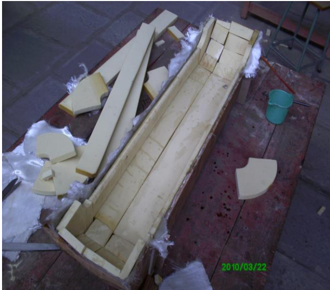
Fig 3.8: placing of foam on mould
